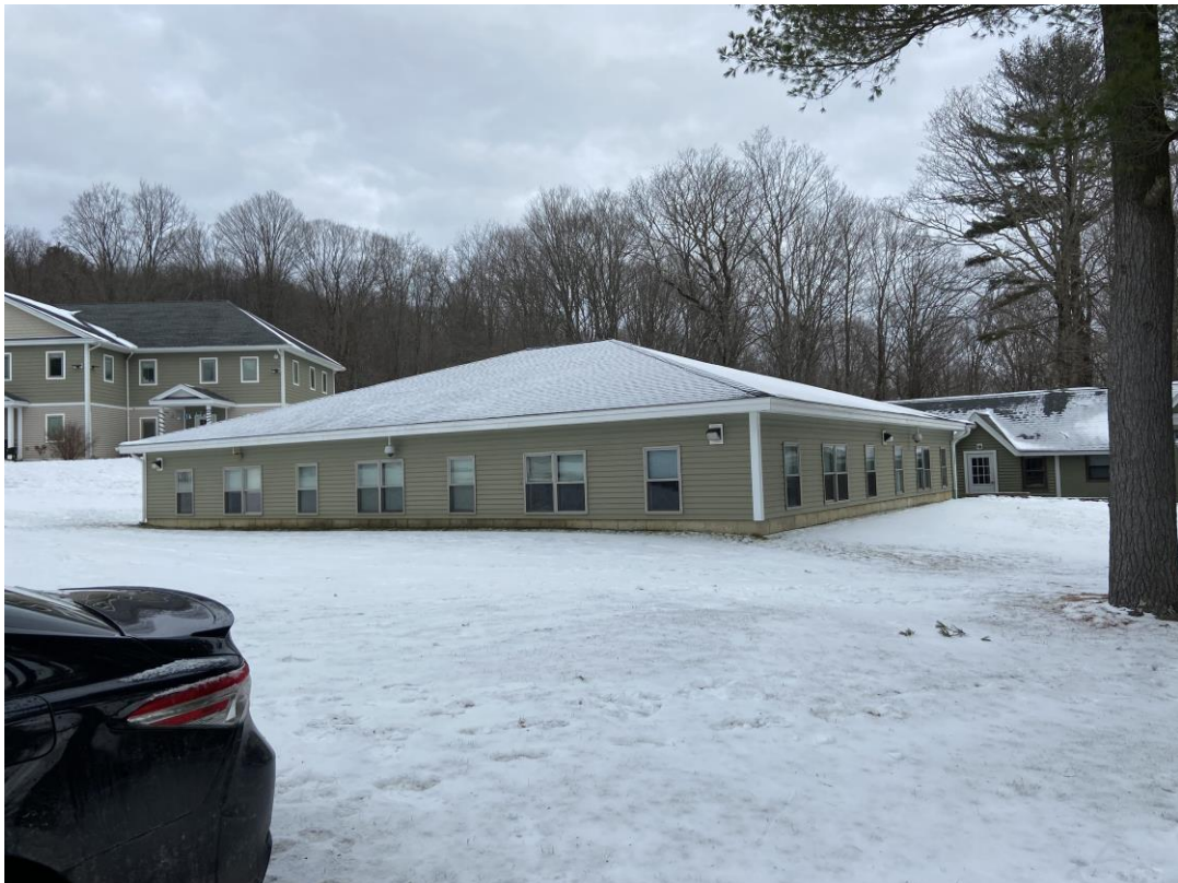
Photo 6: Right-side façade and front façade of existing classrooms/building, facing north-east.
