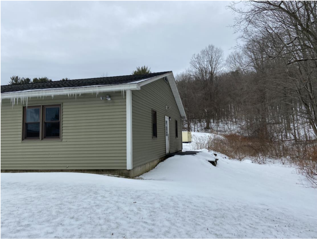
Photo 3: Right-side façade of existing classrooms/building, facing north-west.
