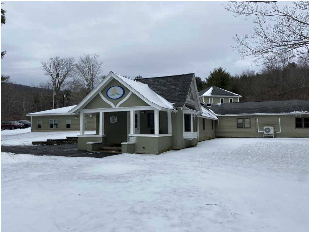
Photo 2: Front façade of existing classrooms/building, facing north-west.
