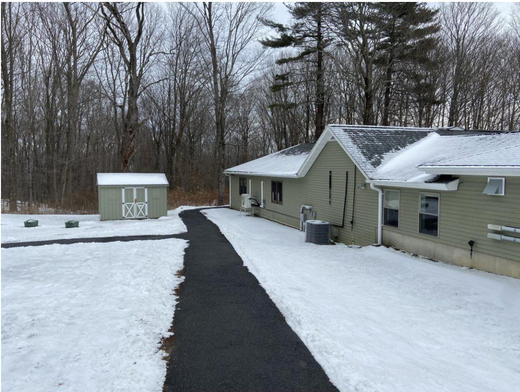
Photo 4: Rear façade of existing classrooms/building, facing east.
