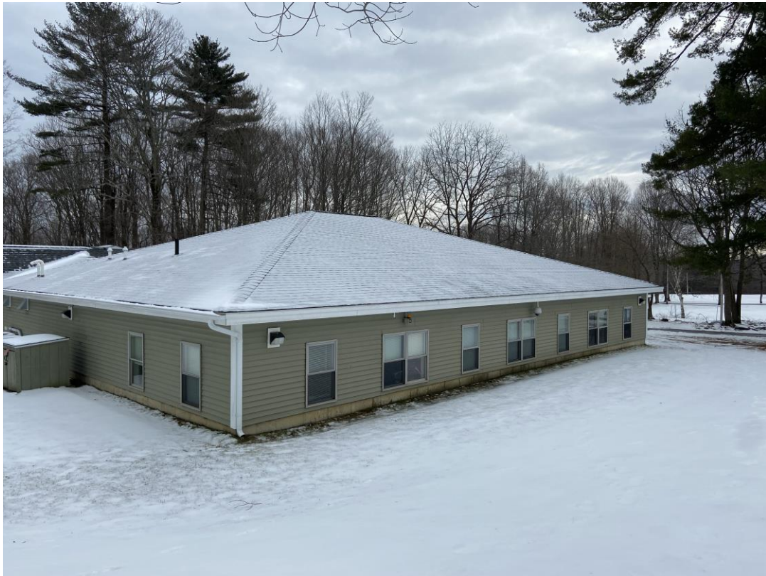
Photo 5: Left-side façade of existing classrooms/building, facing south-east.
