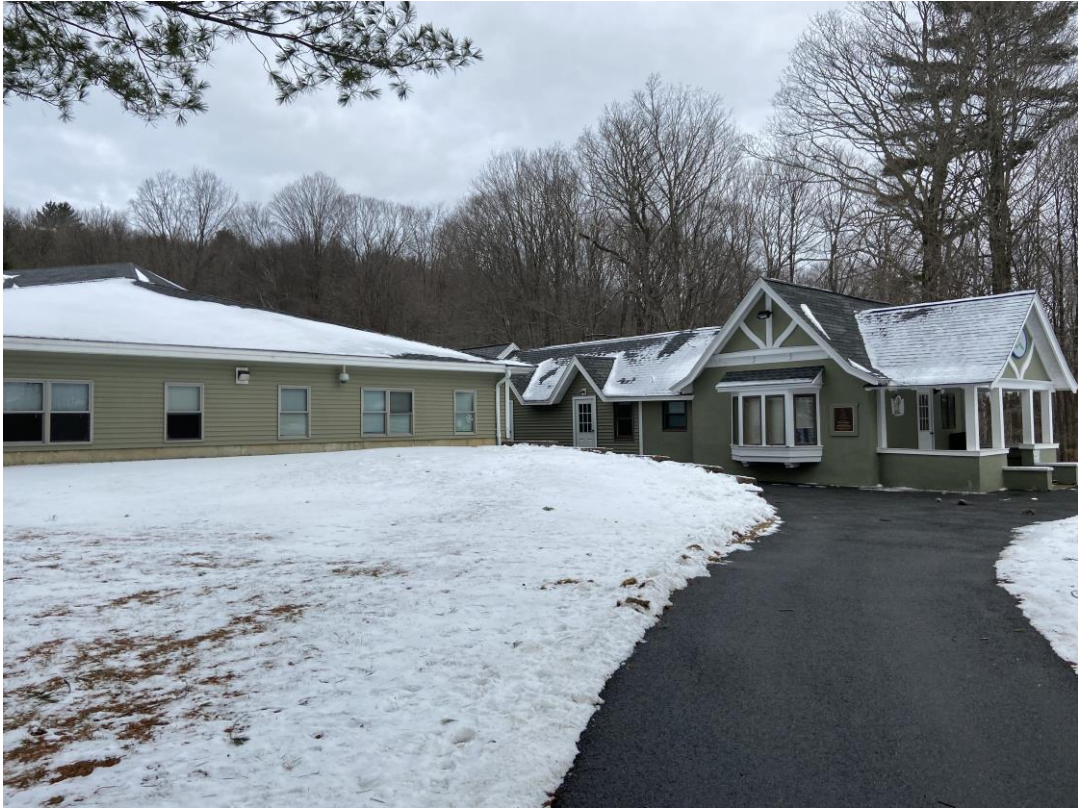
Photo 1: Front façade of existing classrooms/building, facing north.
