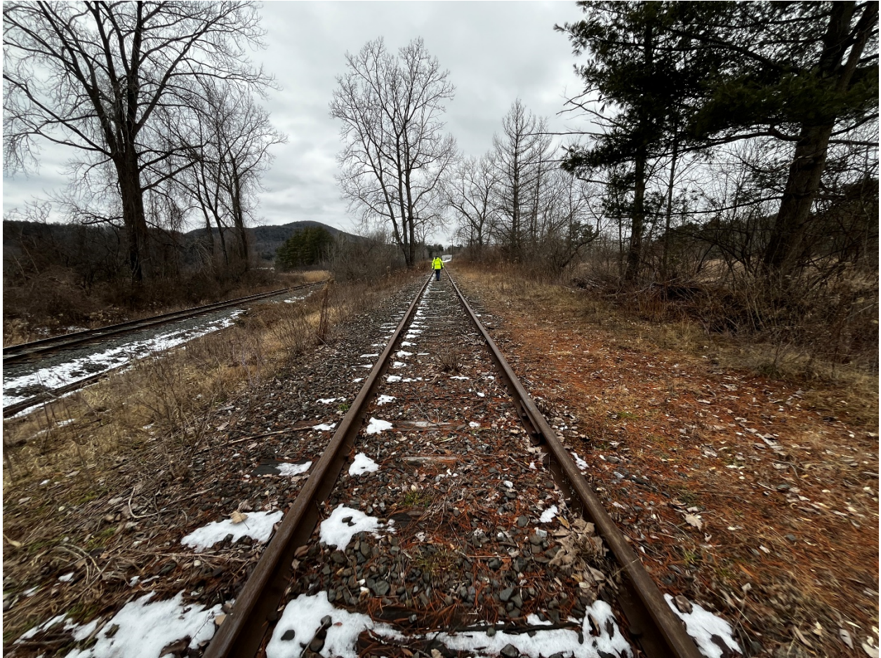
Area surrounding railroad siding to the Onyx Specialty Paper facility located at 1075 Pleasant Street, Lee, along Reach 7D.
