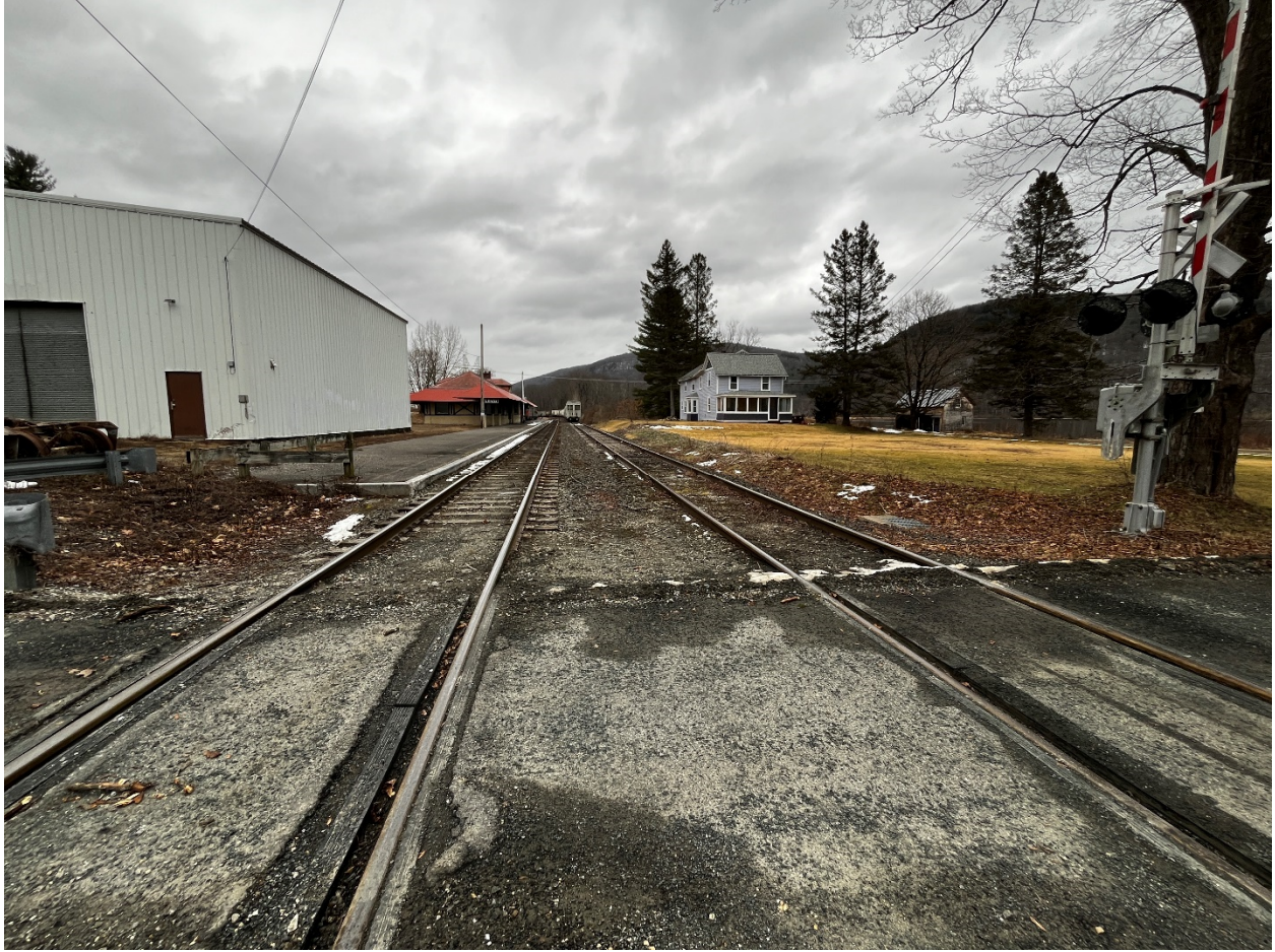
Approximately 0.50 miles of railroad siding adjacent to the Berkshire Scenic Railway Museum in Lenox near Reach 6.
