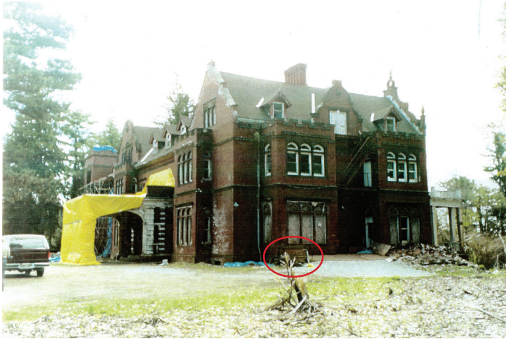
North and west elevations. April, 1998. Masonry work in progress at north elevation. Porte cochere partially covered by a tarp. A remnant of the original terrace wall can be seen at the red circle.
