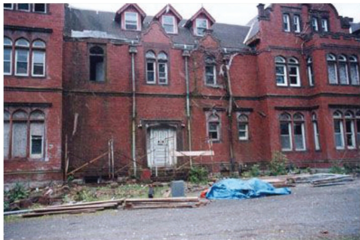
North elevation in 1997. Note the missing shaped gable (over missing sash at second story) allowing damaging water penetration to wall and interior.
