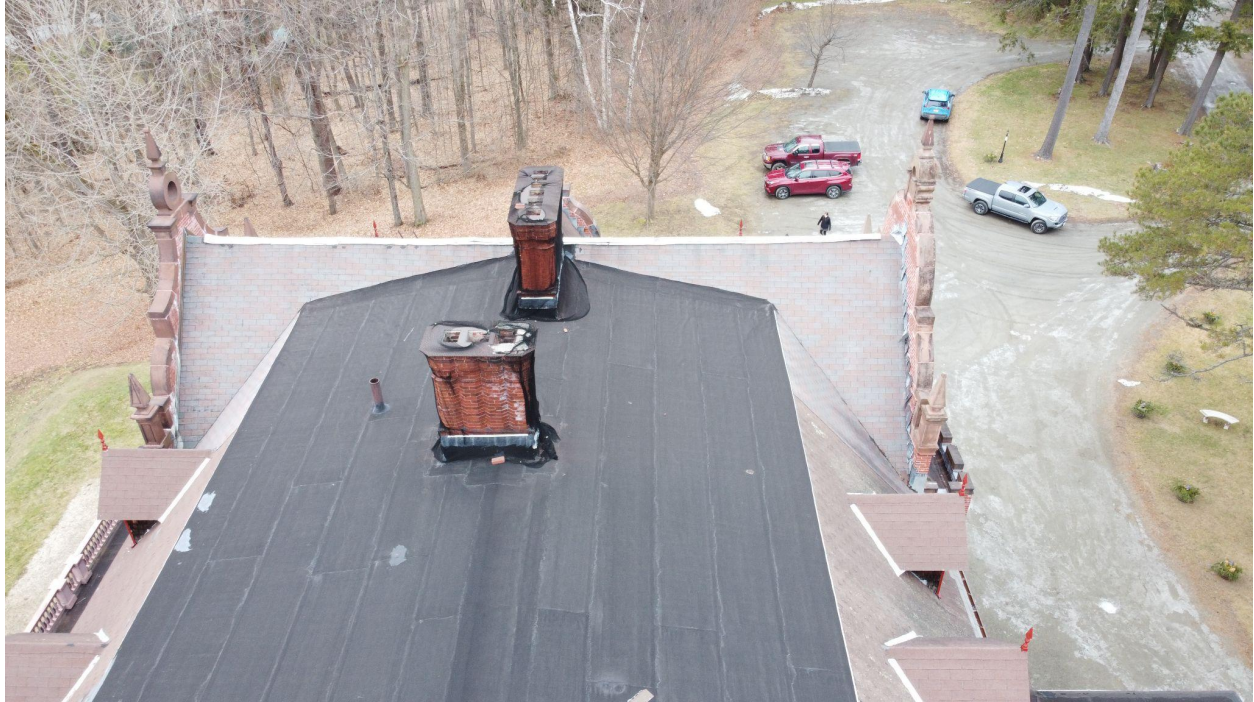
Chimneys on the West side of the roof. Chimneys currently netted for temporary safety.
