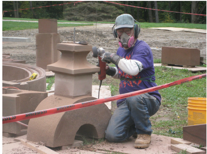
Fabricating finial ornament for south elevation gable peak.
