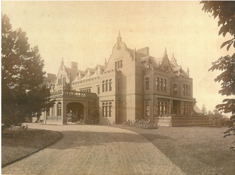
North and west elevations soon after completion in 1893. Note the walled terrace and awning at the west elevation and the upper balustrade at the porte cochere.
