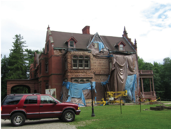
West elevation. July 2007. Rebuilding the west wall.
