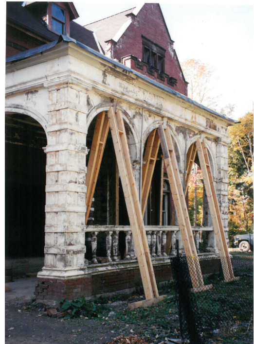
North elevation. Porte cochere shored up prior to disassembly and reconstruction. 1999.
